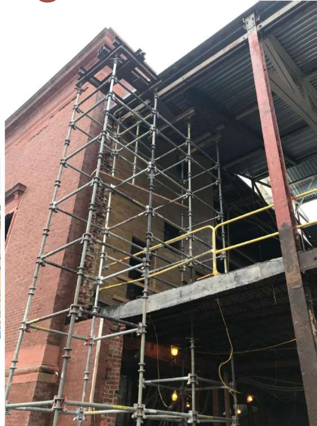
War Memorial Building ( January 2020 ) Post-demolition discovery of structural issues, requiring full facade demolition and structural repairs.
